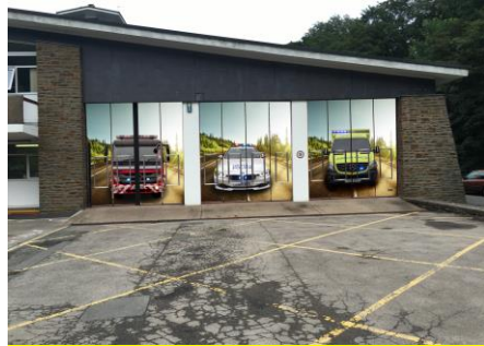
Abertillery Fire Station
